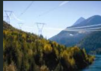
HYDRO ELECTRIC FACILITY
