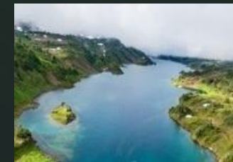
TOM MACKAY TAILINGS FACILITY
