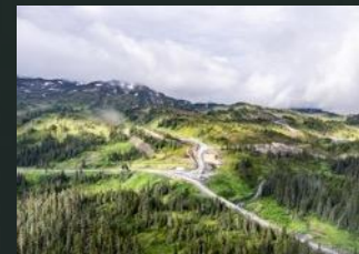
ALL-WEATHER ACCESS ROAD
