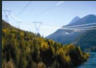
HYDRO ELECTRIC FACILITY
