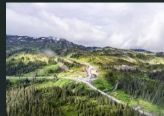
ALL-WEATHER ACCESS ROAD
