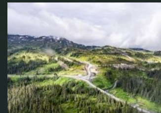
ALL-WEATHER ACCESS ROAD
