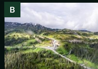
B ALL-WEATHER ACCESS ROAD
